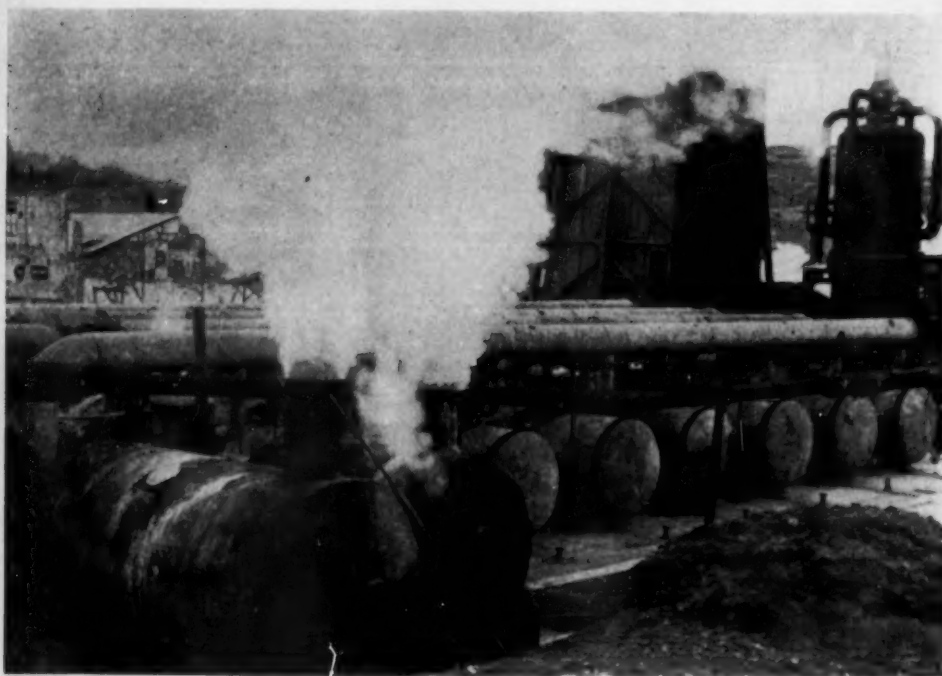
The Chemical plant at Larderello
